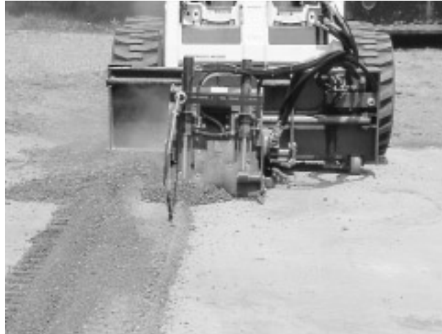
Planer Making Second Pass With Skis Adjusted For Level Cut
